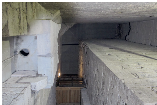
Fig. 9. The isolation shaft surrounding Pikk Hermann Tower (on the right). One of the toilets opening up into the shaft can be seen on the left. Even nowadays as well, access to the tower is by way of a wooden bridge, the base of which is at a height of 9.7 m.
