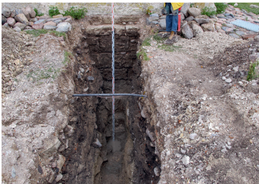
Fig. 6. In excavation XIV from 2012, the southwestern side of the Konventhaus was supported by a previously existing wall that was nearly three metres tall, which protruded in stepped fashion from the wall of the Konventhaus.
