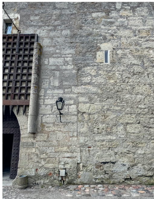
Fig. 7. The vertical joint on the northeastern side of the Konventhaus between Sturvolt Tower (on the right) and the wall of the Konventhaus extends to the lantern. The binding stones protruding from the tower's corner can be seen higher up. The upright limestones placed at the tower's corner near the ground surface suggest that the eastern corner of Sturvolt was restored after the castellum wall had been demolished to a lower height.
