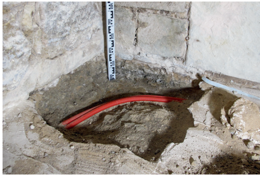
Fig. 8. Test pit no. 19. The foundation of the interior side of the room's northeastern wall (the Konventhaus 's exterior wall, on the right) beside the gate is at an elevation of 3.22 m a.s.l. The room's original floor was situated at more or less the same elevation as the current floor.
