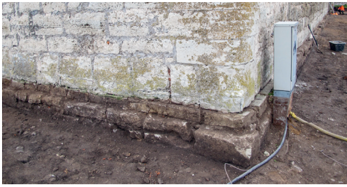
Fig. 5. Southern corner of the Konventhaus. The transition from the right-angled foundation wall to the rounded exterior corners of the Konventhaus with concave facets resembling a pyramid takes place without any intermediate articulation.
