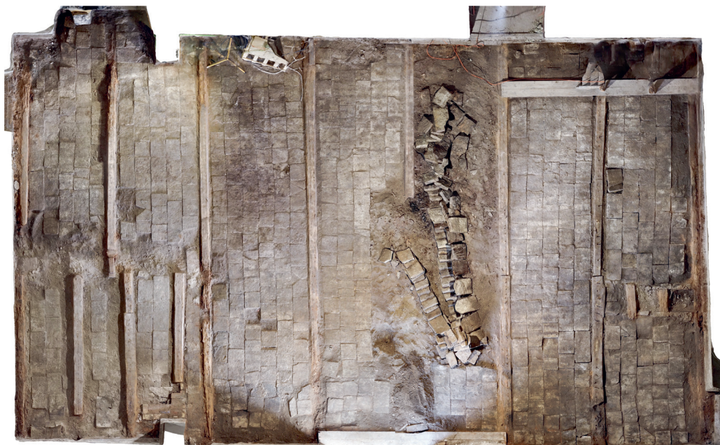
Fig. 15. View of the original 18th-century stone floor of room no. 1 in the harbour storehouse (dimensions 8.9 \times 15 m, ceiling height 5.15 m) that intersects with the foundation beams of the later 19th-century plank floor. Veski Street is at the upper edge of the photograph.
