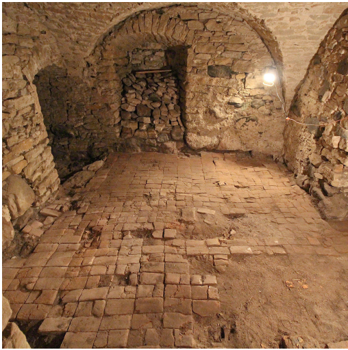
Fig. 2. Tile floor in a basement under the supposed parlatory.
