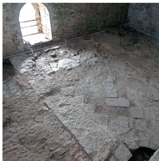
Fig. 5. The floor of square limestone slabs, foundations of a tiled stove, a partition wall and the mantel chimney in the western part of the church.
