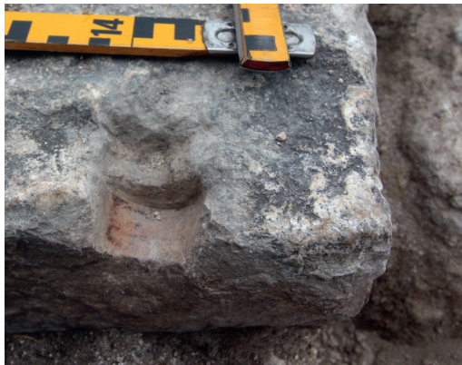
Fig. 9. Recess for the eastern hinge of the drawbridge in the eastern side wall of the gatehouse.
