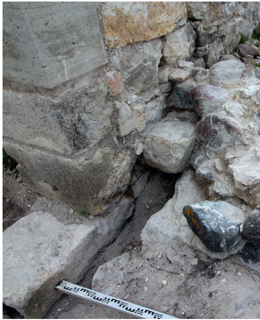
Fig. 8. The eastern chute for the portcullis and the corbel of the initial drawbridge.
