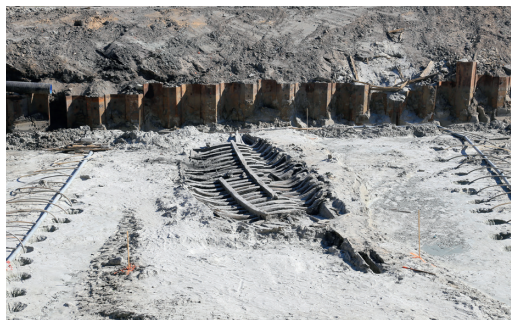
Fig. 3. The excavation pit of wreck Viljo after the well-point dewatering system had been installed.
