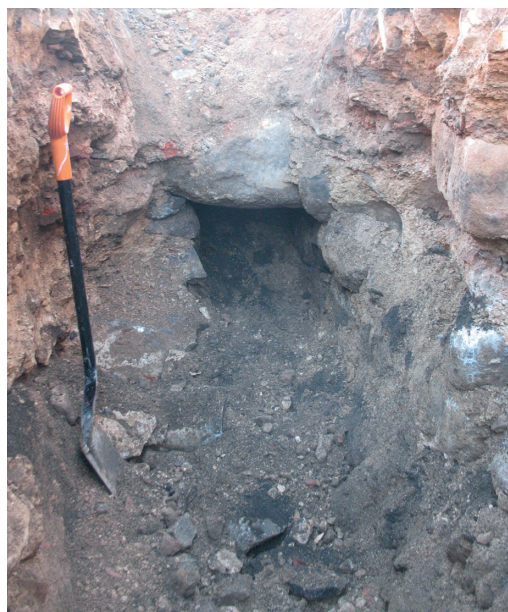
Fig. 3. Gutter in the southern wall of the zwinger of the Riga Gate. View from the west.
