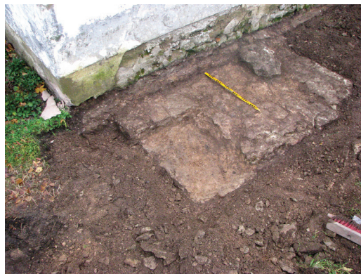
Fig. 5. Foundation of a buttress near the southwestern corner of the nave.
