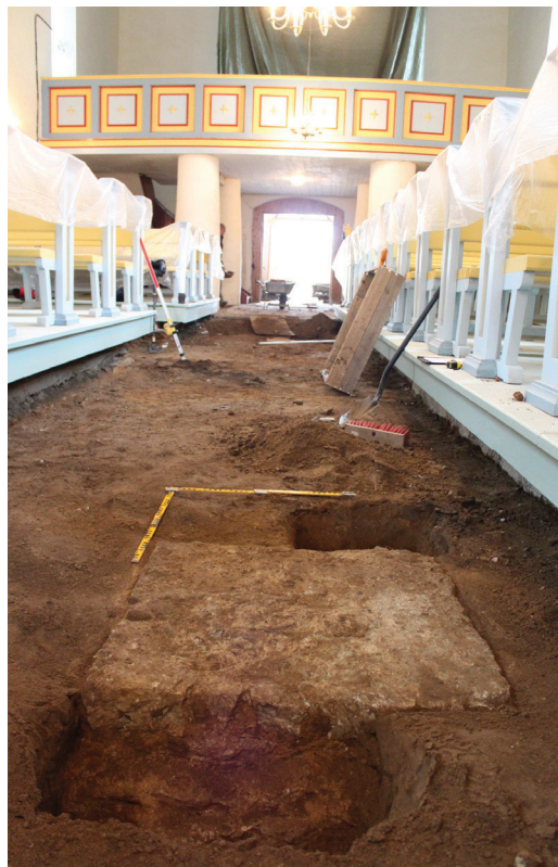
Fig. 6. Foundation of the eastern pillar in the nave.
