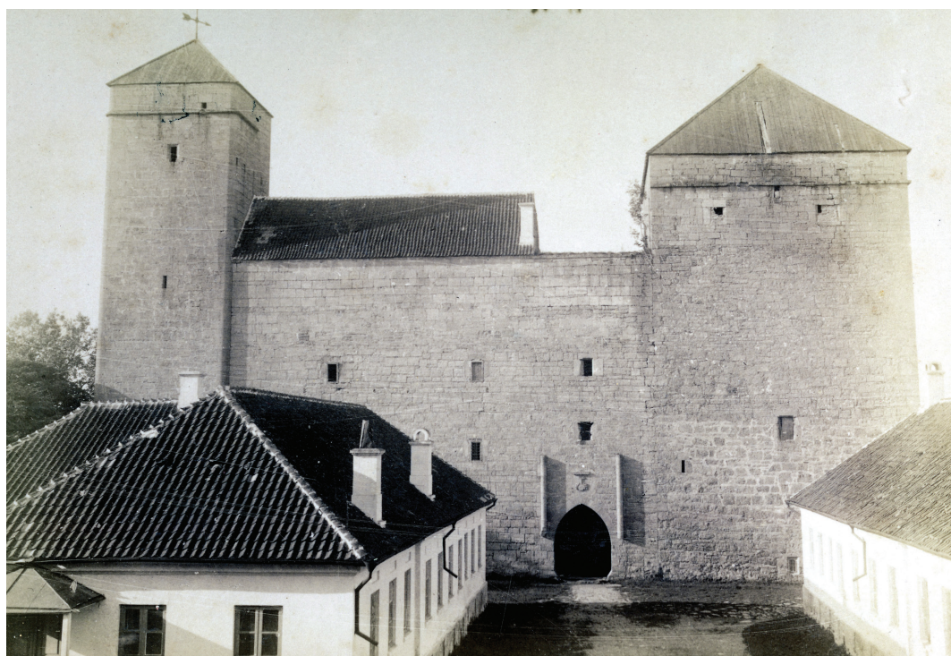
Fig. 2. The Kuressaare Konventhaus in the last quarter of the 19th century, view from the north-east. On the left, the tower of Tall Hermann, on the right, the massive Sturvolt. Binding stones, left during the building of Sturvolt, can be observed quite clearly. On the left in front of the Konventhaus is the officers' building, which was demolished in 1910. On the right the officers' dwelling house, preserved to the present day, can be seen. Today it houses the office rooms of the Saaremaa Museum.
