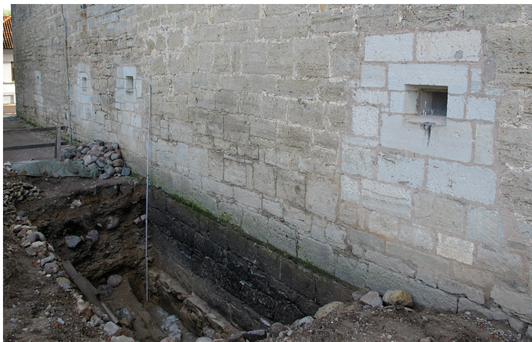
Fig. 3. Excavation XXVII at the junction between the room south-west of Sturvolt and the later north-western wall of the Konventhaus . In the foundation zone uniform stonework without visible building stages can be seen. View from the west.
