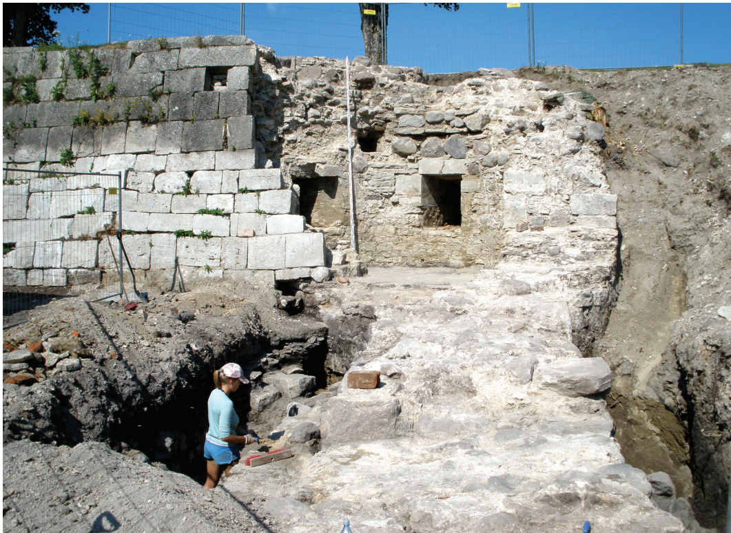
Fig. 9. View of the eastern tower cleared from the north-eastern curtain of the Kuressaare castle, and the surrounding wall demolished to the level of the courtyard ground (excavation II). On both sides of the perch loopholes can be seen, and above them a socket of a beam of an intermediate ceiling. View from south-west.
