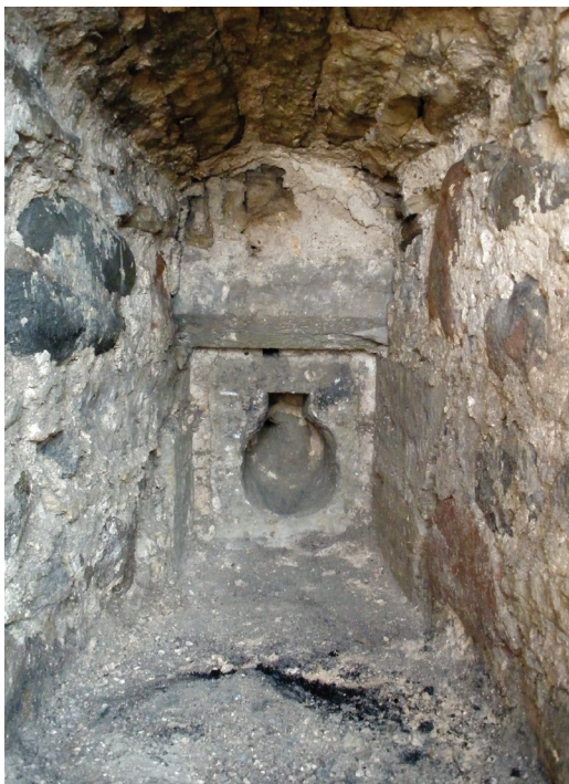
Fig. 11. The three preserved gun ports of the ground floor of the south-east tower were of the key-hole shape, with diameters of 26–31 cm.
