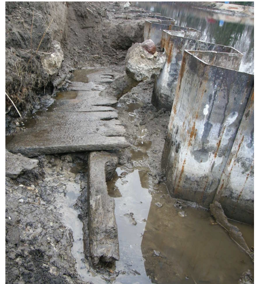
Fig. 10. Supportive construction, composed of horizontal planks and baulks at the southern face of the bastion Luna.
