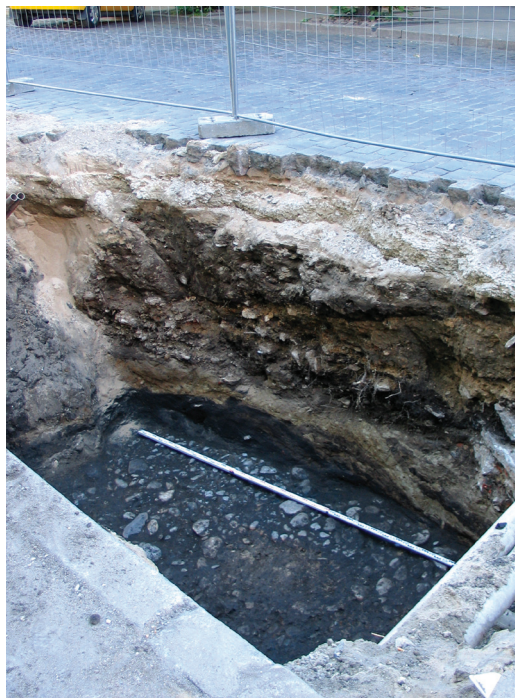
Fig. 4. The 13th century rubble pavement of a road to the Karja gate, under the present-day Suur-Karja street.
