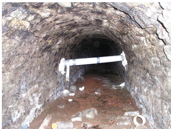
Fig. 13. Limestone water conduit for the drinking water from Lake Ülemiste.
