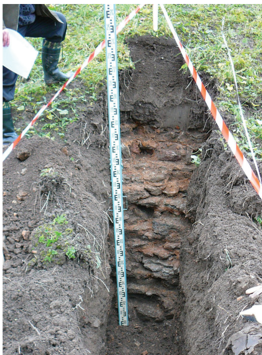
Fig. 5. Breast-wall foundation in the test pit of the 5th ravelin.
