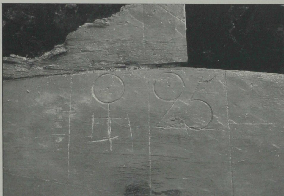
Fig. 5. Technological markers on one of the ship's frames.
