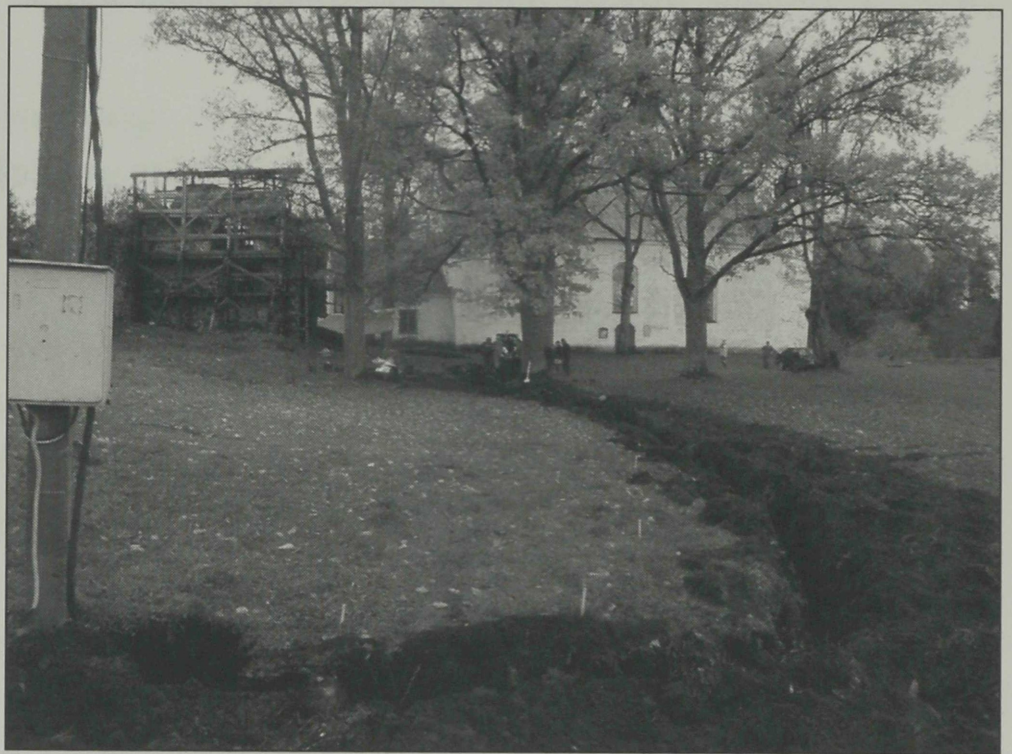
Fig. 1. The beginning of the first trench along the northern wall of the outer bailey of Karksi castle.
