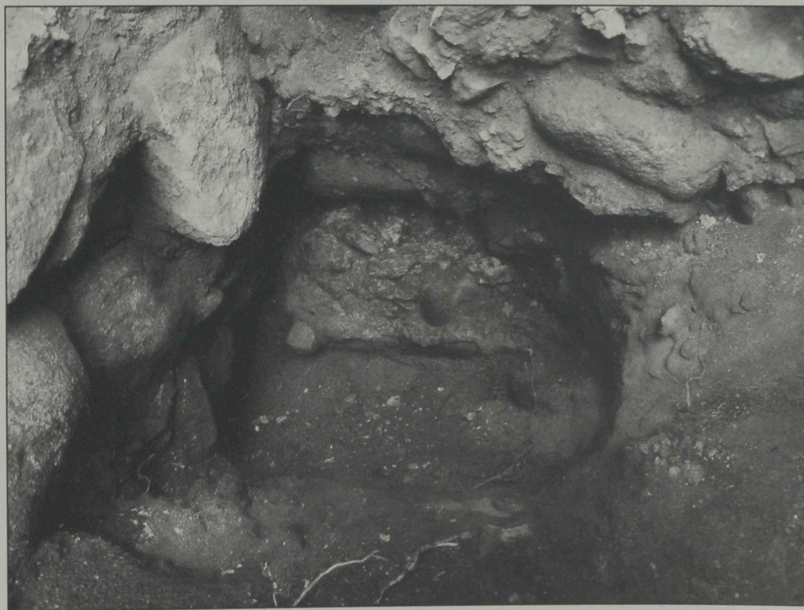
Fig. 4. The foundation of small pebbles joined with abundant lime mortar in the test-pit on the eastern side of the gate building.
