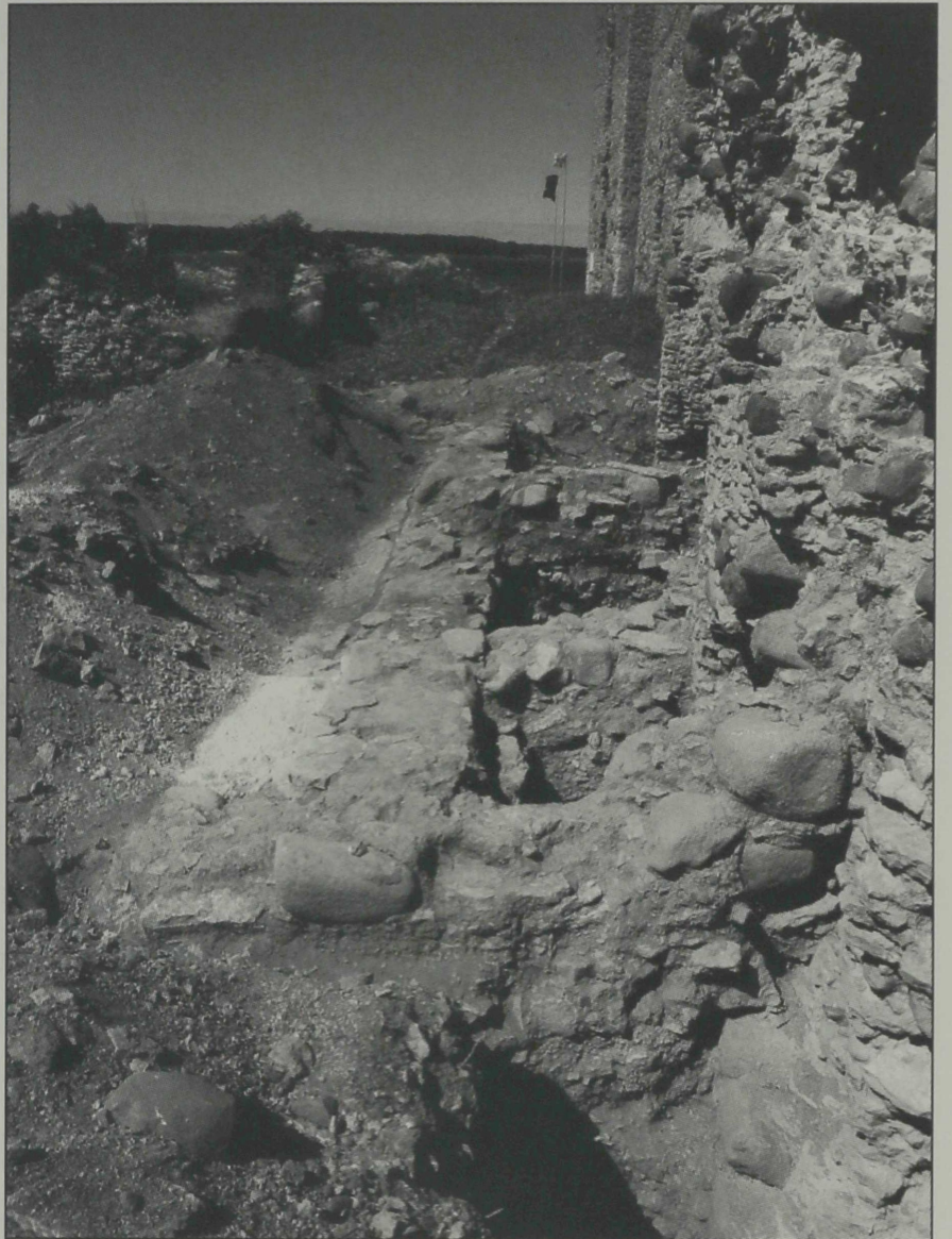
Fig. 3. Foundation of the auxiliary building of the tavern on the southern side of the gate building.
