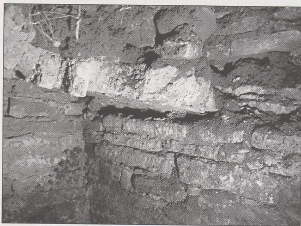
Fig. 3. Northwest corner of the chamber. Note the shallow arch of the brick vault, groove on the northern wall and gap in the corner.
