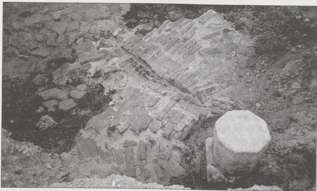
Fig. 4. The collapsed vaults. View from SE.
