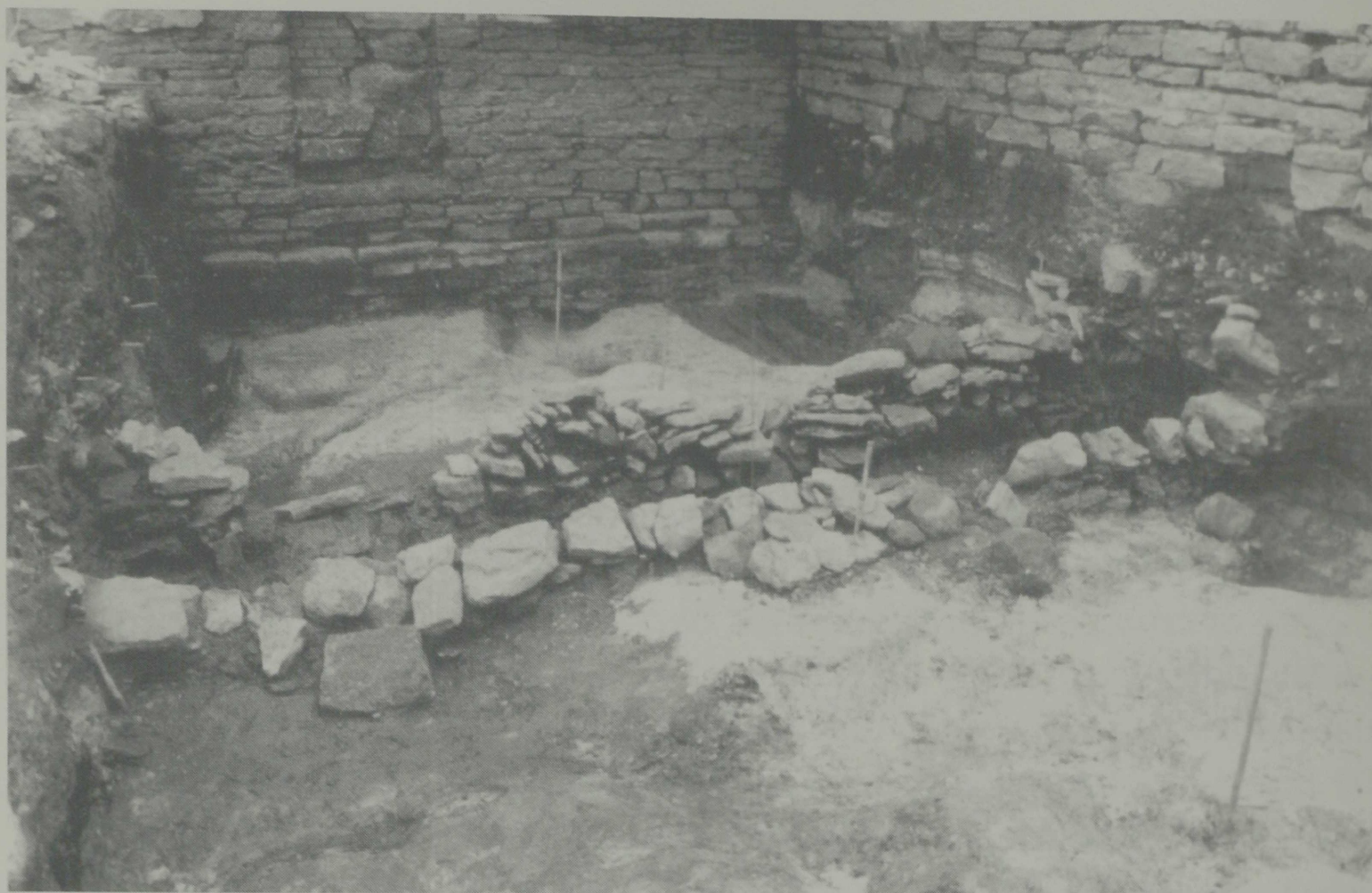
Fig. 4. Sewage canal stoned with limestone slabs.
