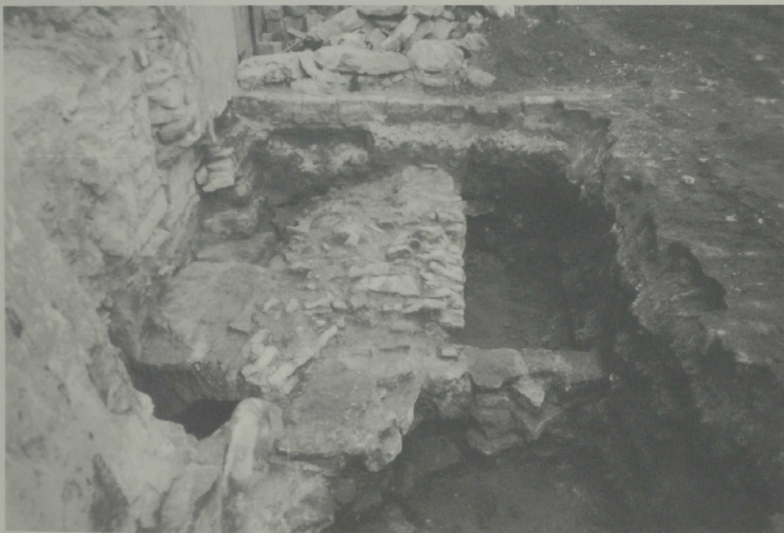
Fig. 10. Lavatory constructions in the yard of Raeapteek. View from the east.
